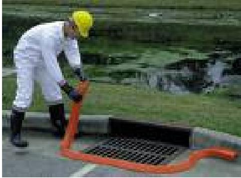
1. **Containment Booms** – Protective barriers can be placed around a storm drain in order to prevent water from entering the drain. They are normally used in order to prevent wastewater from entering a stormwater drain and to pool the wastewater around drain for later collection. However, one potential problem with booms is that they can be ineffective or less effective when the storm drain is located at the bottom of a slope or if there is a large amount of wastewater generated.
